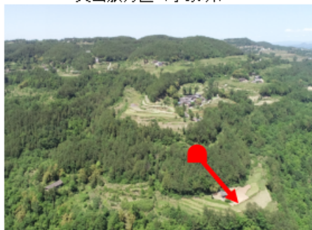
灵山隧道终点
